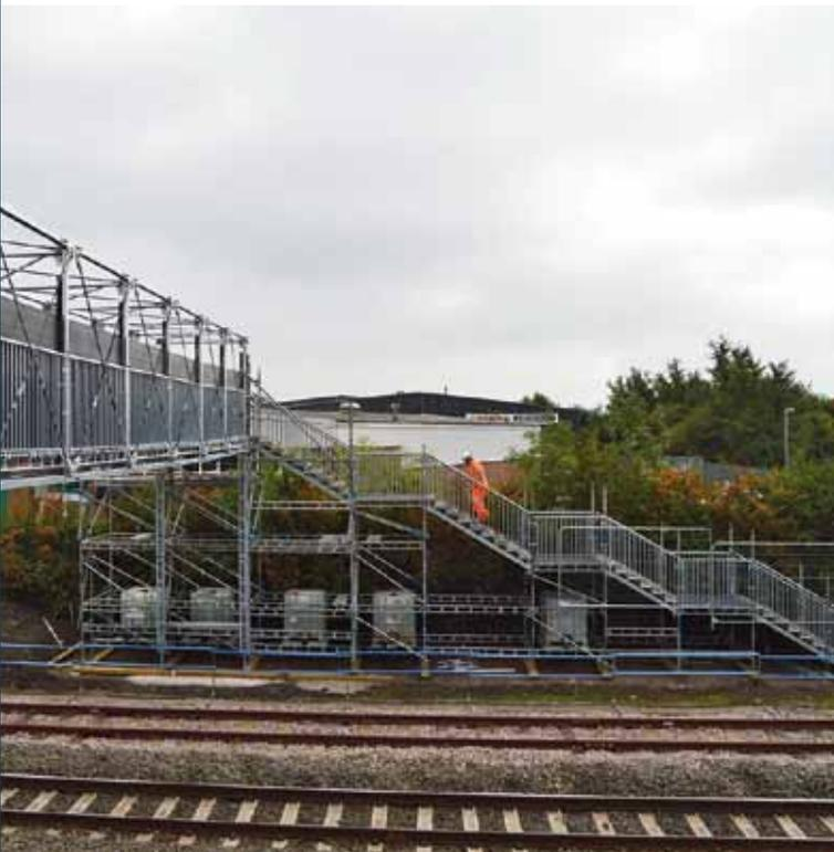
Stair towers provide a safe and quick access and egress to the workplace. The modular design and lighter components make the stairs quick and simple to erect.
